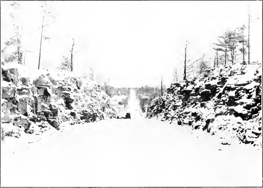
Rock Cut and Bridge, Highway No. 7, Marmora Looking East.
